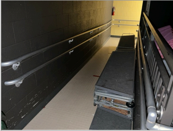
ACCESSIBLE INTERIOR RAMP
