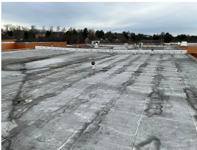
5 - PRIMARY ROOF OVERVIEW
