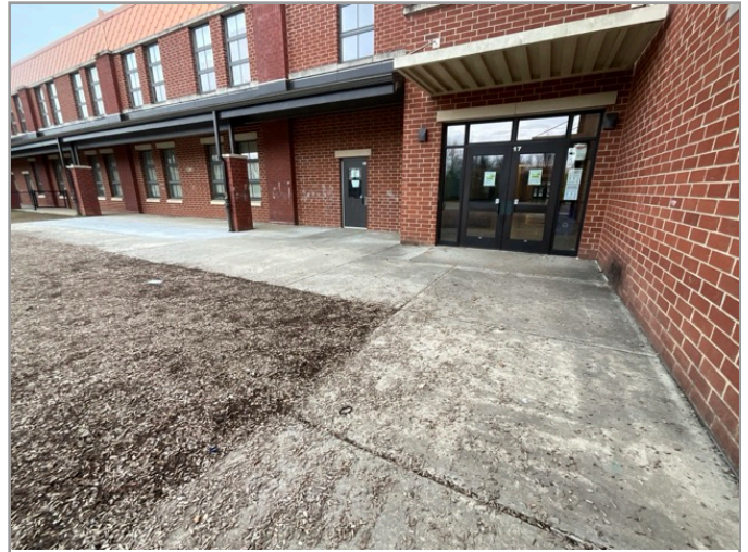
ACCESSIBLE ROUTE TO PLAYGROUND
