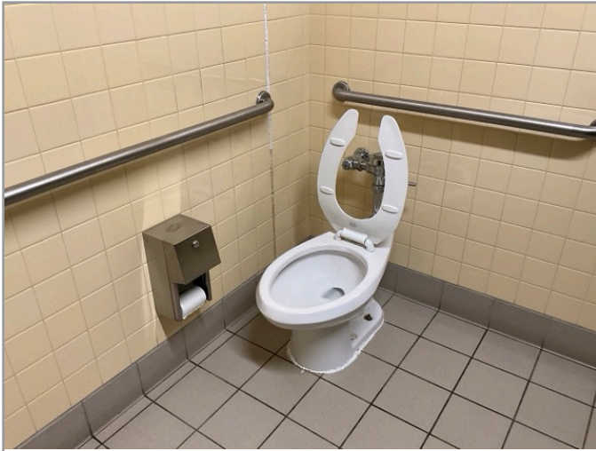
TOILET STALL OVERVIEW
